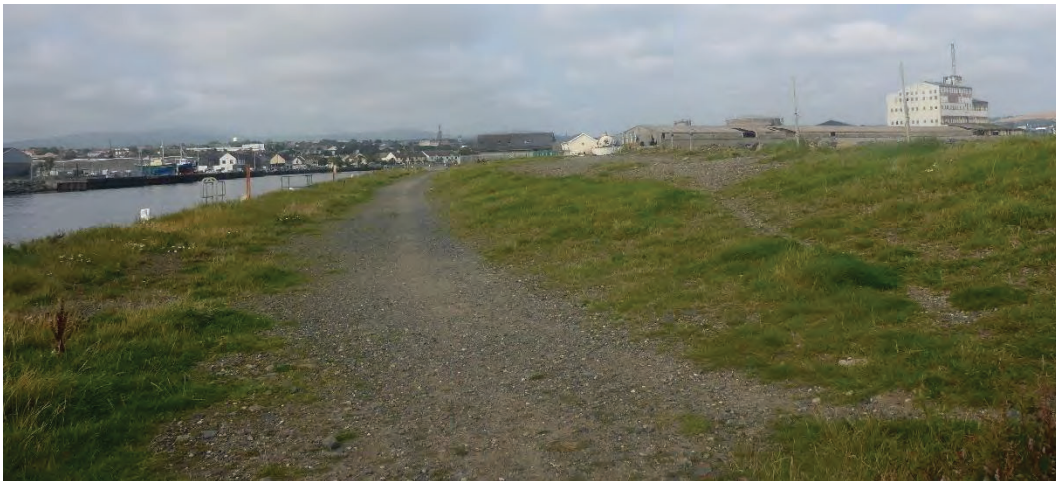
Figure 2.24: Site Compound 5 (SC5) looking westwards.
