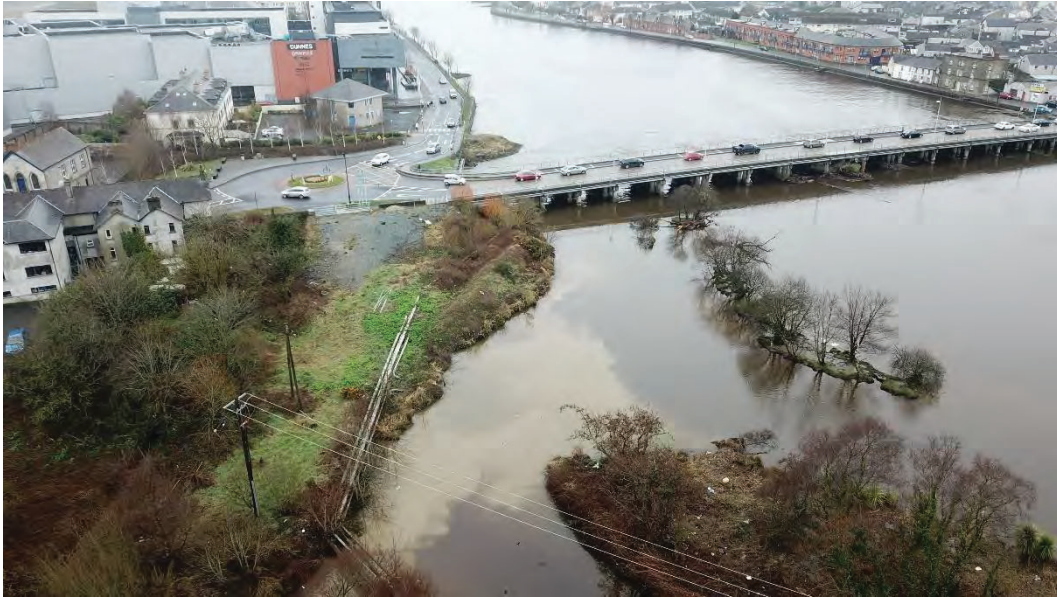
Figure 2.21: Site Compound 3 (SC3)
