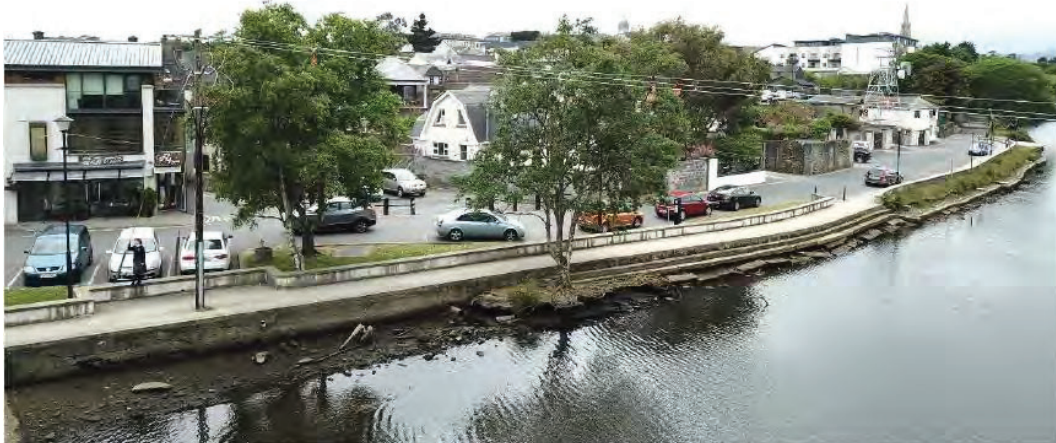
Figure 2.6: River Walk (viewed from the river channel looking westward) Source: Google Maps
