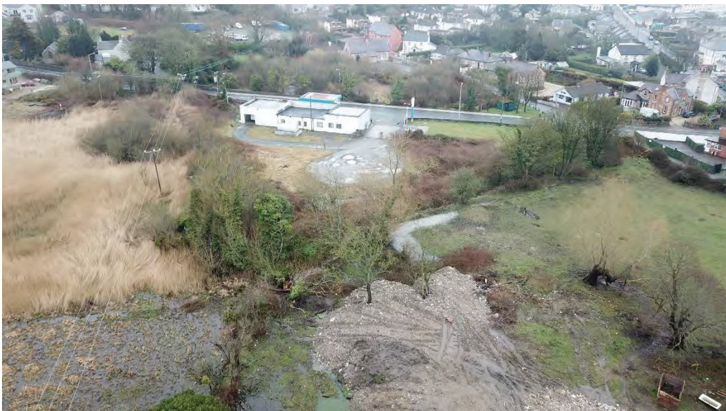
Figure 2.18: Site Compound 1 (SC1)
