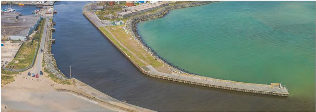
Figure 2.23: Site Compound 5 (SC5)
