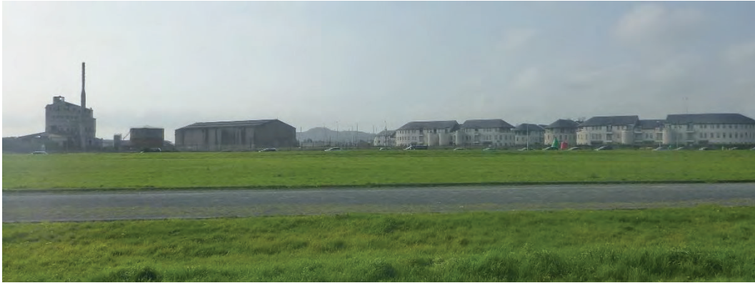
Figure 2.19: Site Compound 2 (SC2)
