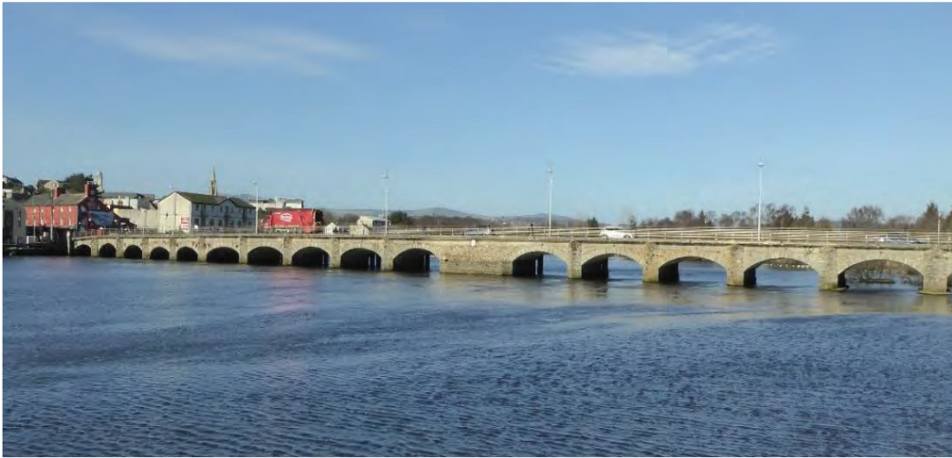
Figure 2.9: Arklow Bridge (viewed from downstream on North Quay. Looking westward) Source: Google Maps
