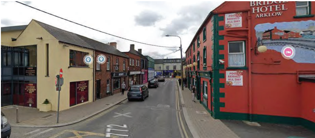
Figure 2.12: Bridge Street (View from Arklow Bridge looking southwards) Source: Google Maps
